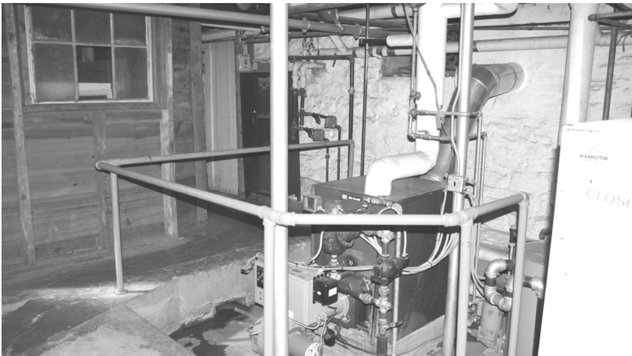
FIGURE 155. View northwest in furnace room. (T. Jones, NPS-SERO-CR, 2004)
