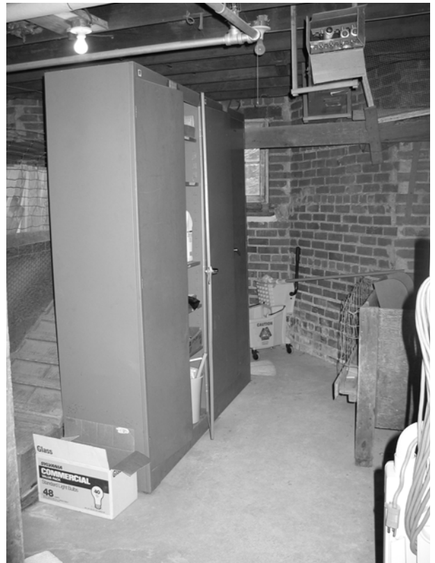
FIGURE 154. View southeast in Room 010. (T. Jones, NPS-SERO-CR, 2004)
