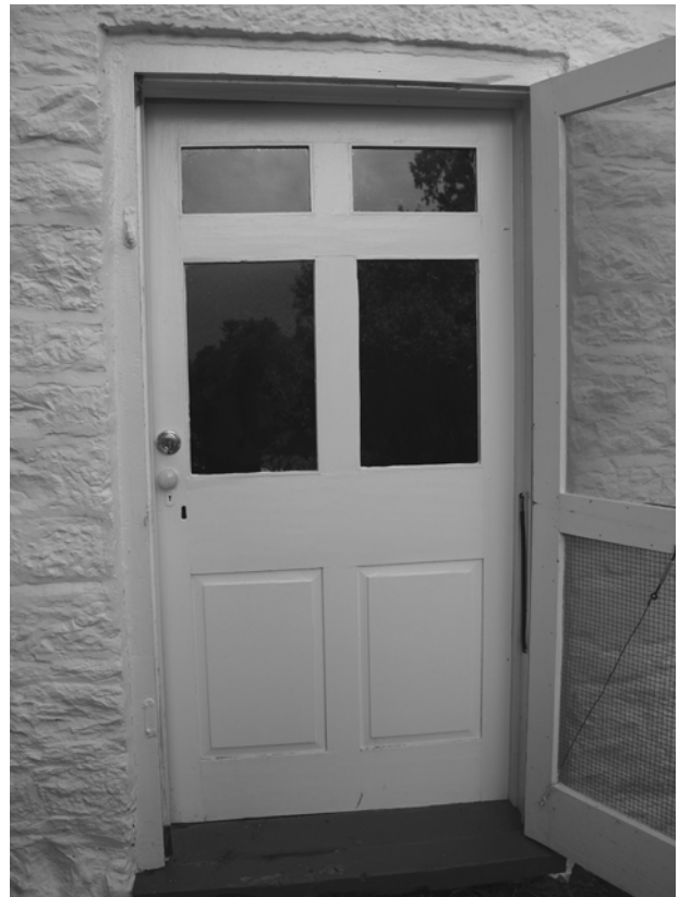
FIGURE 124. View of Door D-1, one of the house's original doors (c. 1838), altered by the Sandburgs in 1945. (T. Jones, NPS-SERO-CR, 2004)
