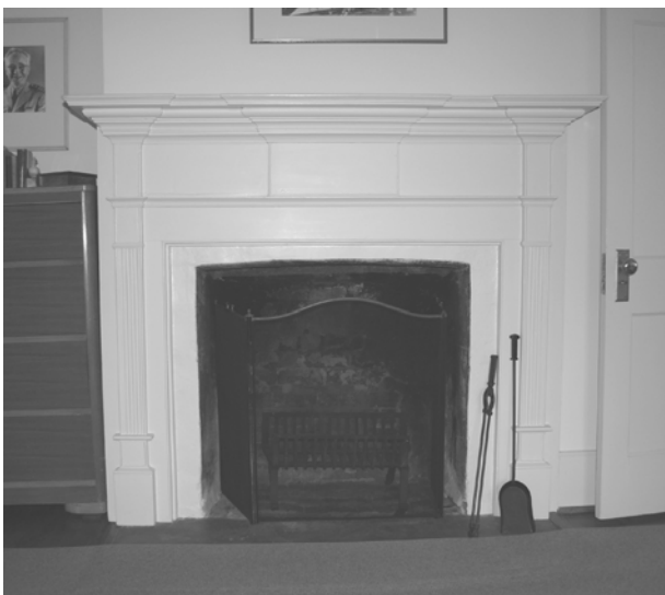
FIGURE 169. View of mantel in Mrs. Sandburg's Bedroom (121). A similar mantel was removed from the house, probably from Room 113 or 118, and is now stored in the wood shed. (T. Jones, NPS-SERO-CR, 2004)
