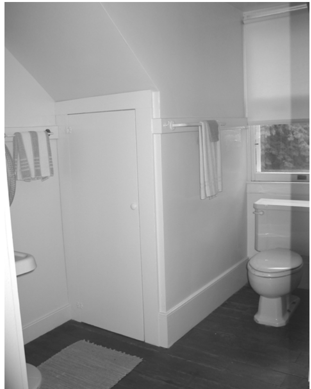
FIGURE 211. View southeast in Room 217. (T. Jones, NPS-SERO-CR, 2004)
