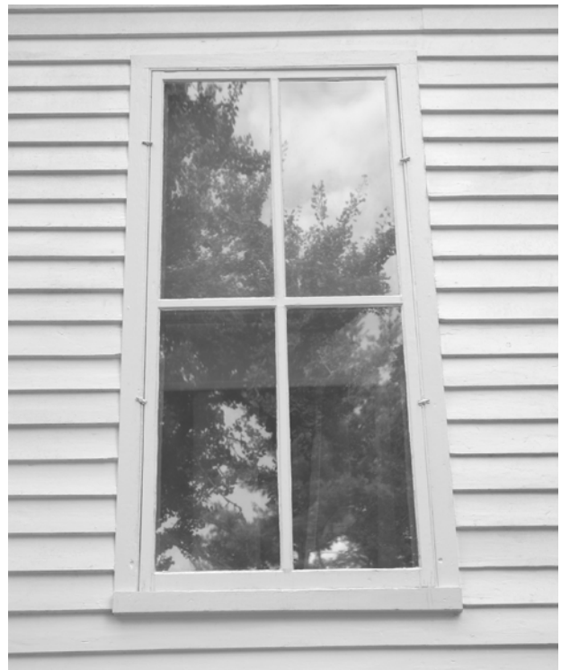
FIGURE 120. View of window (W-36), with original narrow beaded casing and thick sills used at openings on the sides of the original house. (T. Jones, NPS-SERO-CR, 2004)
