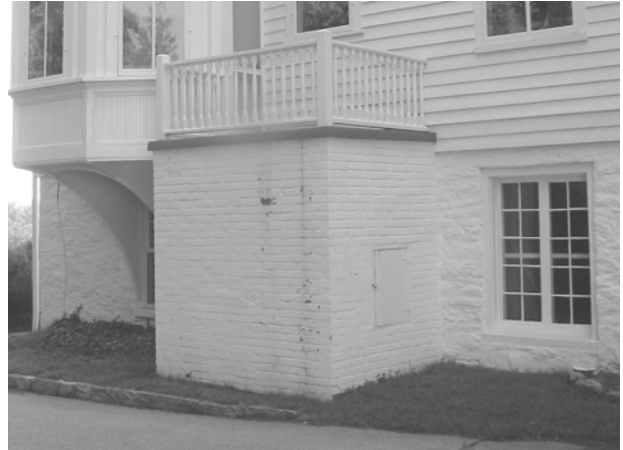
FIGURE 139. View of West Porch. (T. Jones, NPS-SERO-CR, 2004)
