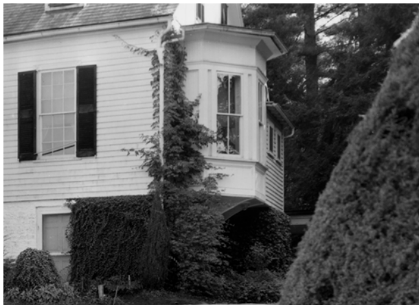
FIGURE 83. View of west end of house, c. 1938, with bathroom addition just visible beyond the bay window and a glimpse of the carport beyond that. (CARL3001/23/03P, photo by Bayard Wooten, Carolina Collection, University of North Carolina)
