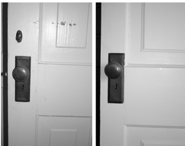
FIGURE 163. View of late nineteenth-century, four-panel doors D-43 (left) and D-26 (right) (T. Jones, NPS-SERO-CR, 2004)
