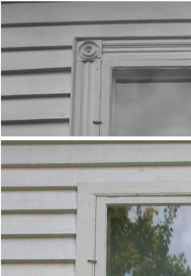
FIGURE 126. View of original (1838) exterior window casings. (T. Jones, NPS-SERO-CR, 2004)
