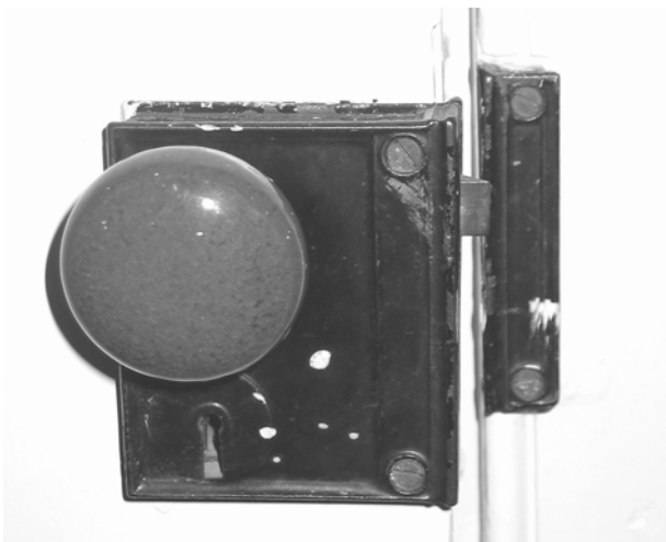
FIGURE 199. View of typical late-nineteenth century rim lock in Sandburg's Study (201). (T. Jones, NPS-SERO-CR, 2004)
