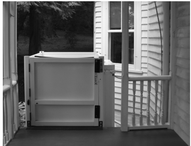
FIGURE 135. View of lift to East Porch..(T. Jones, NPS-SERO-CR, 2004)
