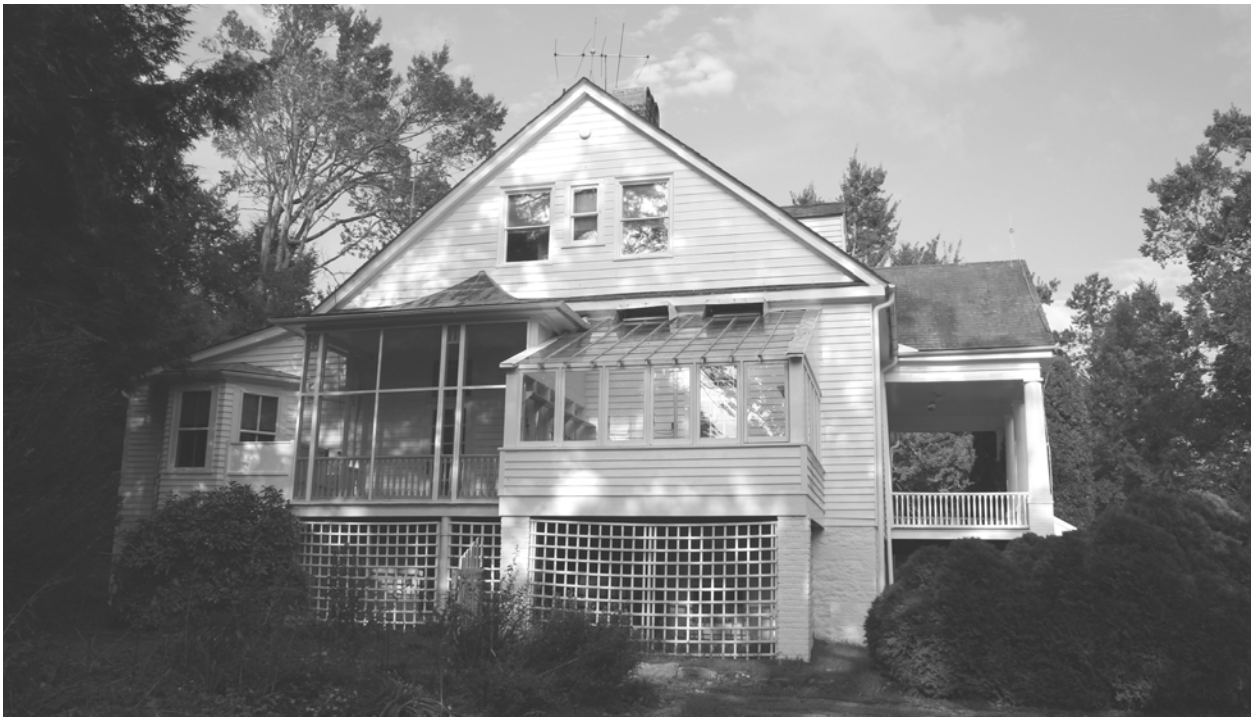
FIGURE 110. View of reconstructed conservatory and east end of house. (T. Jones, NPS-SERO-CR, 2004)
