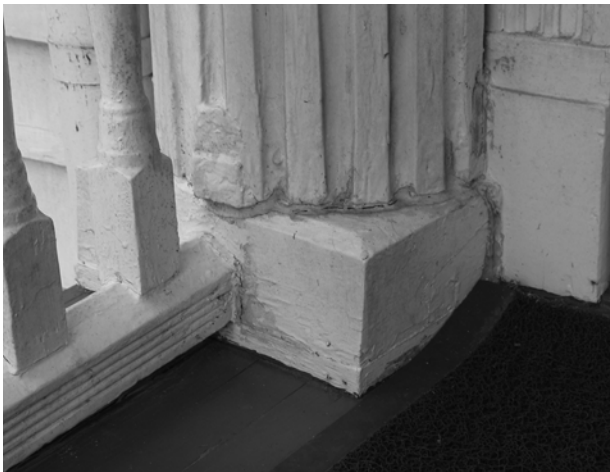
FIGURE 132. View of pilaster plinth on Portico. (T. Jones, NPS-SERO-CR, 2004)
