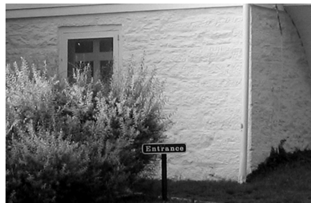
FIGURE 109. View of foundation at northwest corner of original house.(T. Jones, NPS-SERO-CR, 2004)
