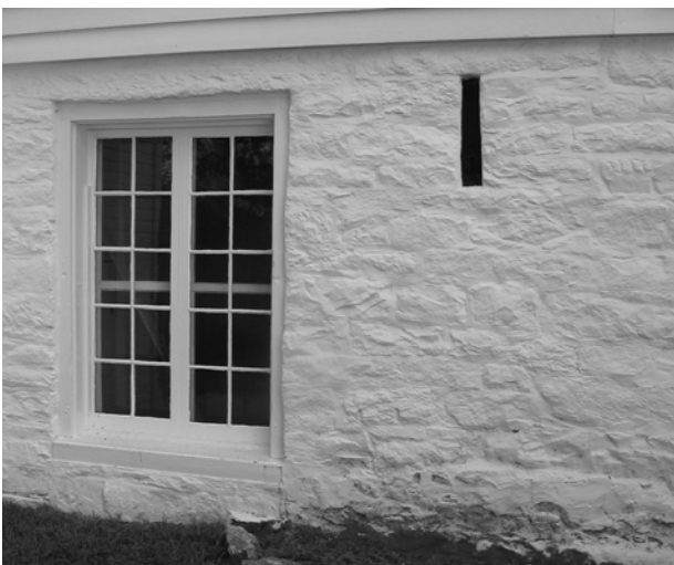
FIGURE 123. View of window W-13, which was originally a door opening, and the adjacent embrasure. (T. Jones, NPS-SERO-CR, 2004)
