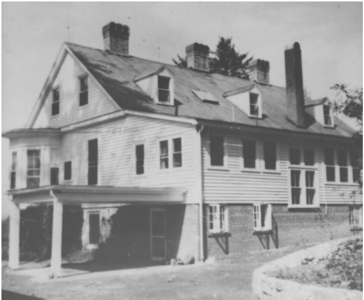
FIGURE 85. View of rear and west end of house in 1946 or early 1947. Aga stove chimney had not yet been built and the foundation remains unpainted. (CARL3000/15/26P)
