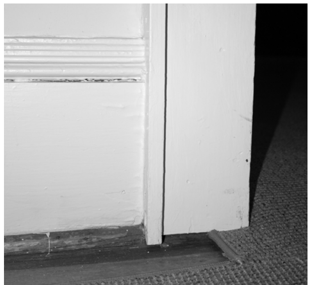
FIGURE 166. View of baseboard and casing typical of 1924 additions. (T. Jones, NPS-SERO-CR, 2004)
