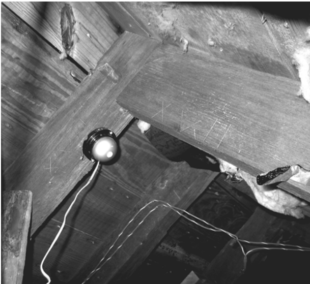
FIGURE 115. View of typical connection of rafters in main roof. Note inscribed Roman numeral XVII on face of right-hand rafter. (T. Jones, NPS-SERO-CR, 2004)
