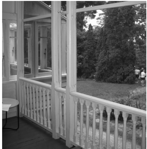
FIGURE 134. View of original posts and balustrades (c. 1890) on East Porch..(T. Jones, NPS-SERO-CR, 2004)
