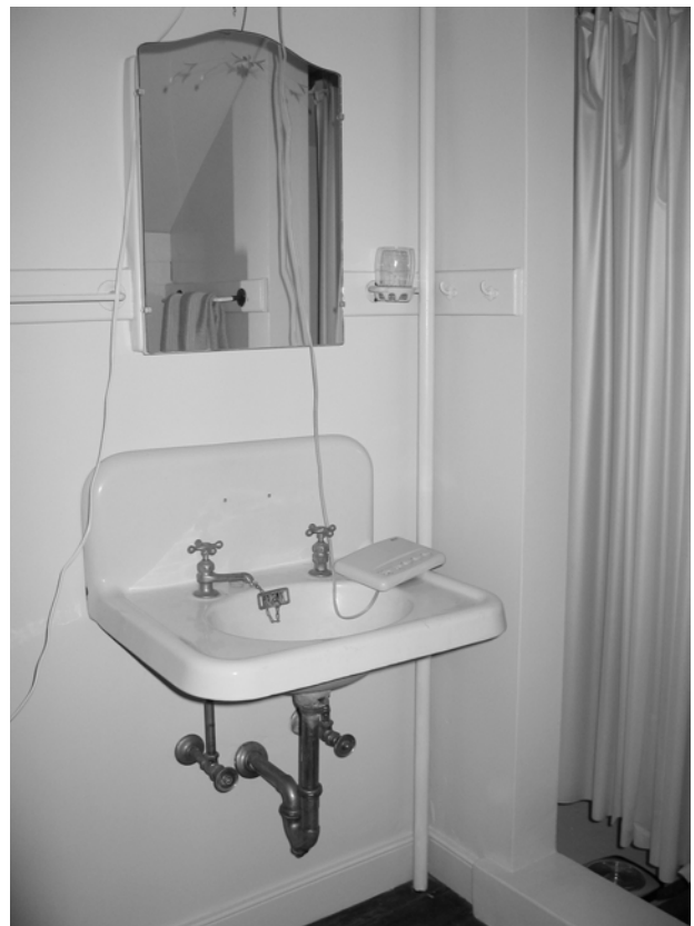
FIGURE 212. View northeast in Room 217. (T. Jones, NPS-SERO-CR, 2004)
