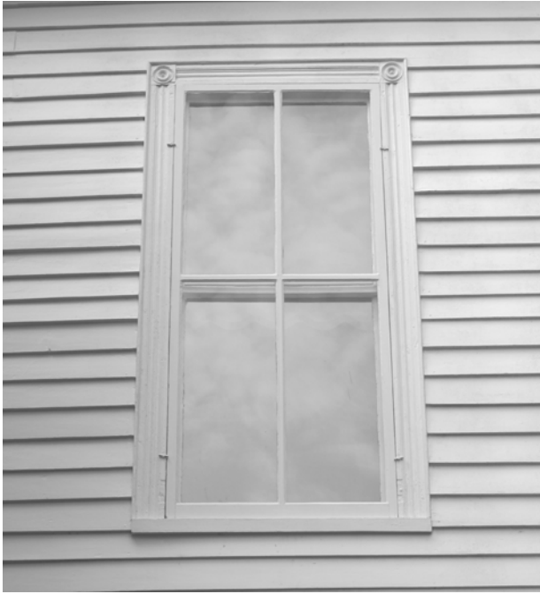
FIGURE 118. View of Window W-36, showing typical original casing and sill. Nine-over-nine muntins have been removed from original sash. A four-light, exterior storm sash is installed at the opening in this image. (T. Jones, NPS-SERO-CR, 2004)
