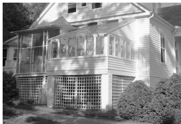
FIGURE 136. View of East Porch and Conservatory..(T. Jones, NPS-SERO-CR, 2004)
