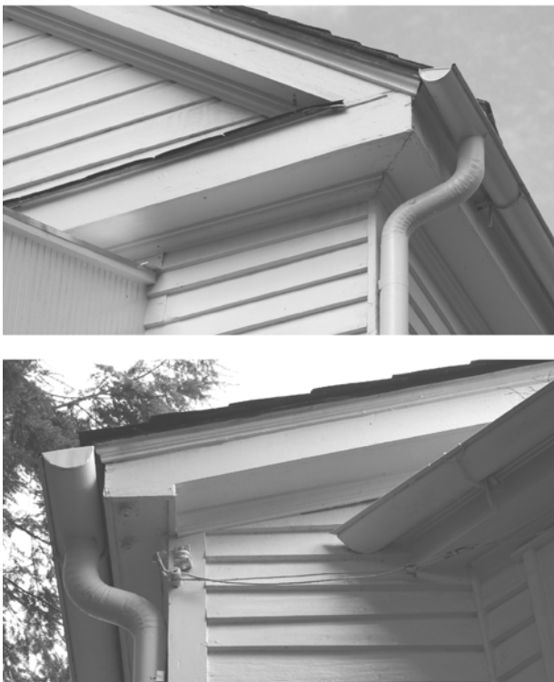
FIGURE 127. View of typical eaves on original house, top, and on rear addition, bottom. (T. Jones, NPS-SERO-CR, 2004)
