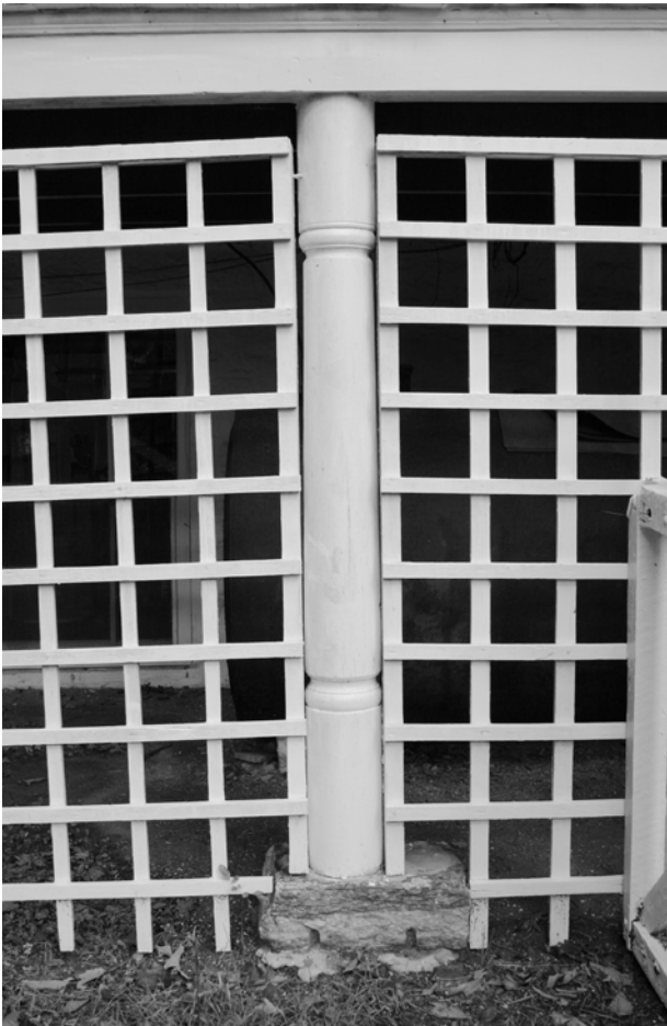
FIGURE 138. View of lattice under East Porch..(T. Jones, NPS-SERO-CR, 2004)
