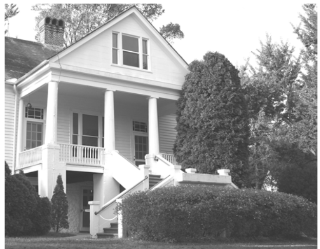
FIGURE 130. View of Portico.(T. Jones, NPS-SERO-CR, 2004)
