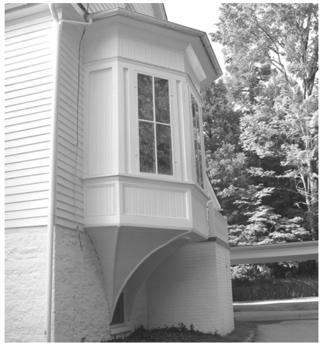
FIGURE 128. View of west bay window.(T. Jones, NPS-SERO-CR, 2004)
