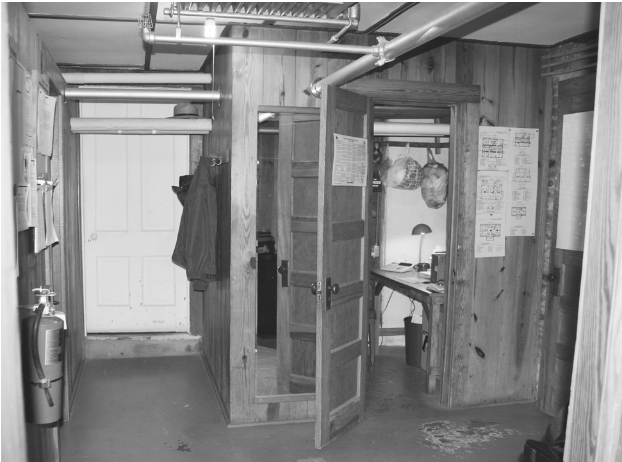
FIGURE 152. View west in Room 005, with view into Room 006. (T. Jones, NPS-SERO-CR, 2004)
