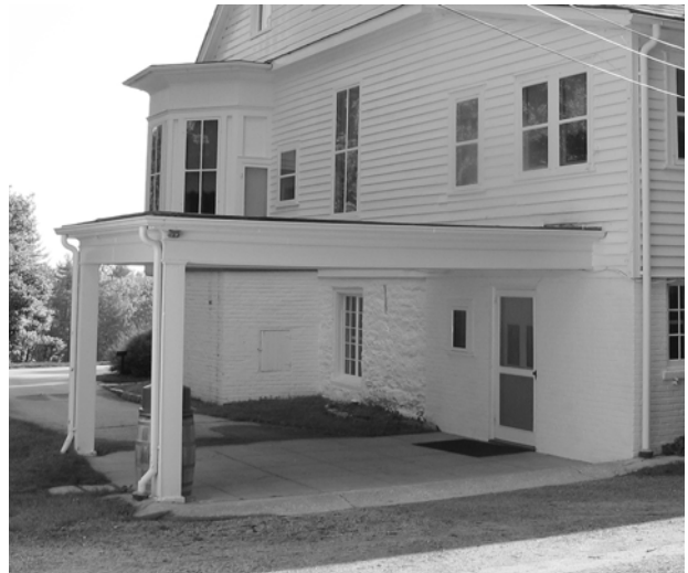
FIGURE 140. View to northeast of porte cochere. (T. Jones, NPS-SERO-CR, 2004)
