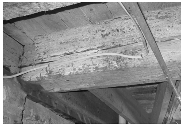
FIGURE 112. View of hand-hewn beam in Room 018. (T. Jones, NPS-SERO-CR, 2004)
