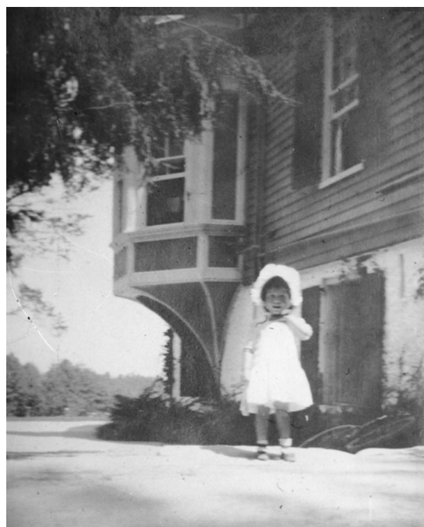
FIGURE 76. Smyth grandchild at west end of Main House, showing west bay and exposed waste lines and vent stacks for the lavatories in the Rooms 118 and 121. (CARL3001/01/32P)
