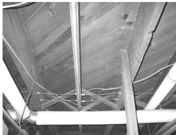
FIGURE 113. View of typical, cross-braced, floor joists and diagonally laid sub-floor in rear addition. (T. Jones, NPS-SERO-CR, 2004)
